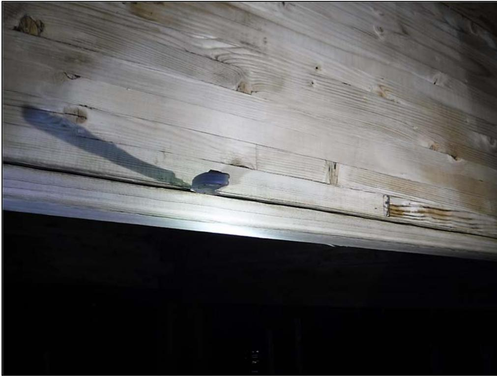
**Photo 10 – Delamination of the bottom lamination at valley glulam beam 1 between purlins L and K indicated by the knife inserted 4” into the separation.**
