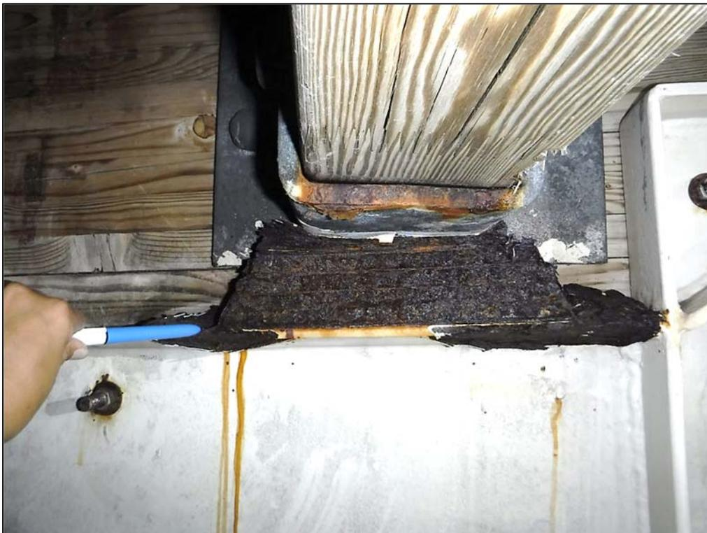
Photo 18 – Corroded shims at valley glulam beam 13 and purlin L.
