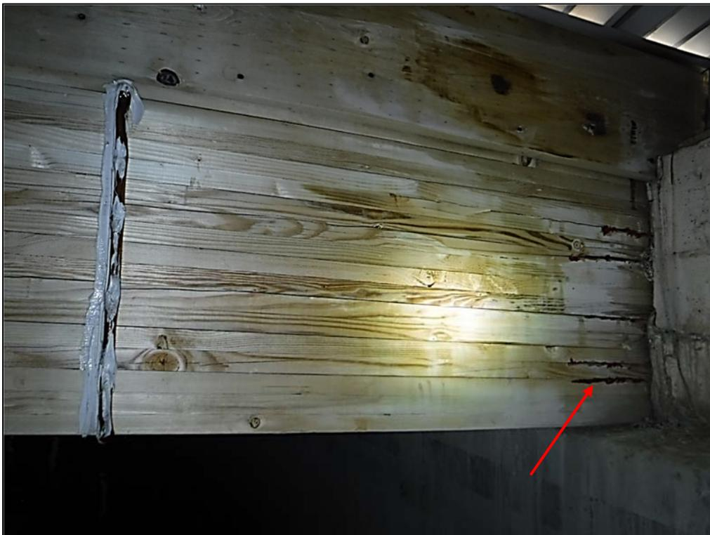
**Photo 11 – Valley glulam beam 17 at cmu wall. The red arrow points to seams where epoxy has been injected as a repair attempt.**
