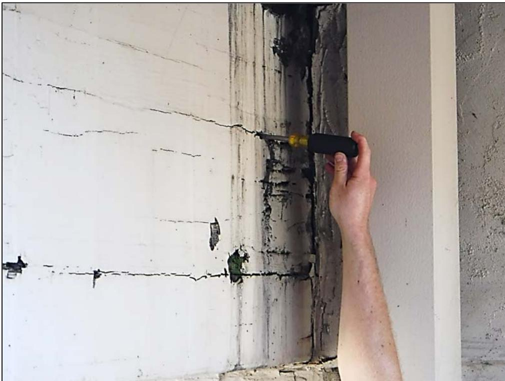
**Photo 15 – Close up of typical dry rot on exterior valley glulam beam 21; beam is very soft with up to 4" penetration near the cmu wall interface.**
