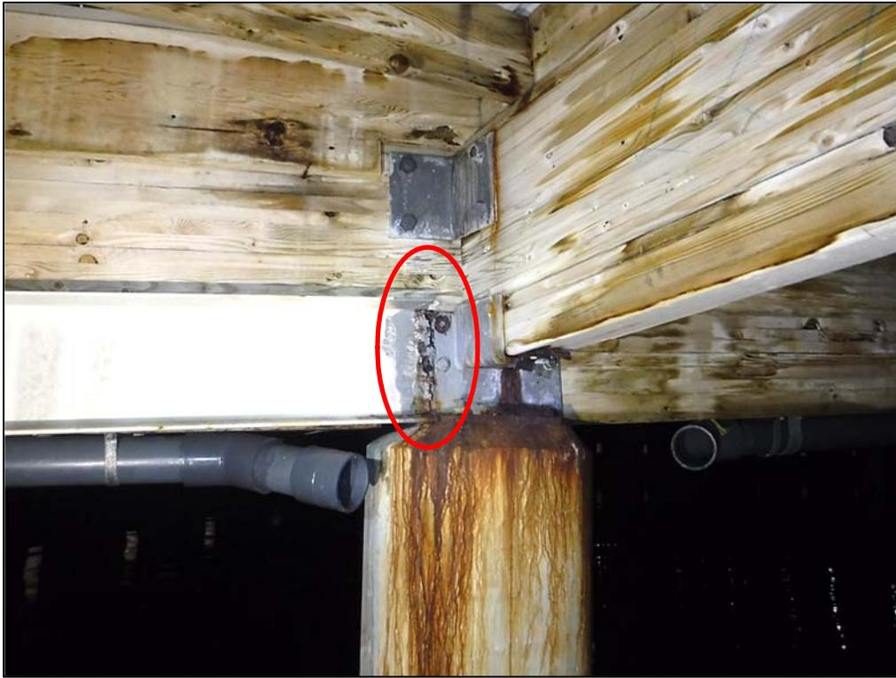
Photo 17 – Welded connection corrosion at valley glulam beam 13 and purlin J.
