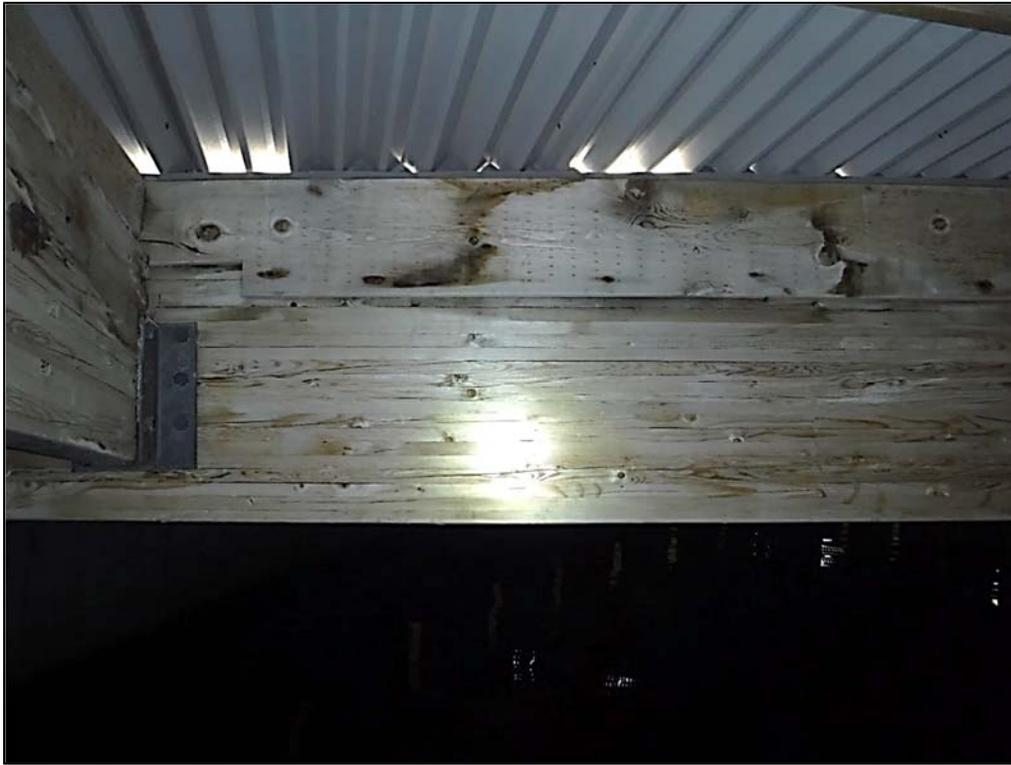
Photo 12 – Check at valley glulam beam 21 between purlin L and K, detail shown in Photo 13.
