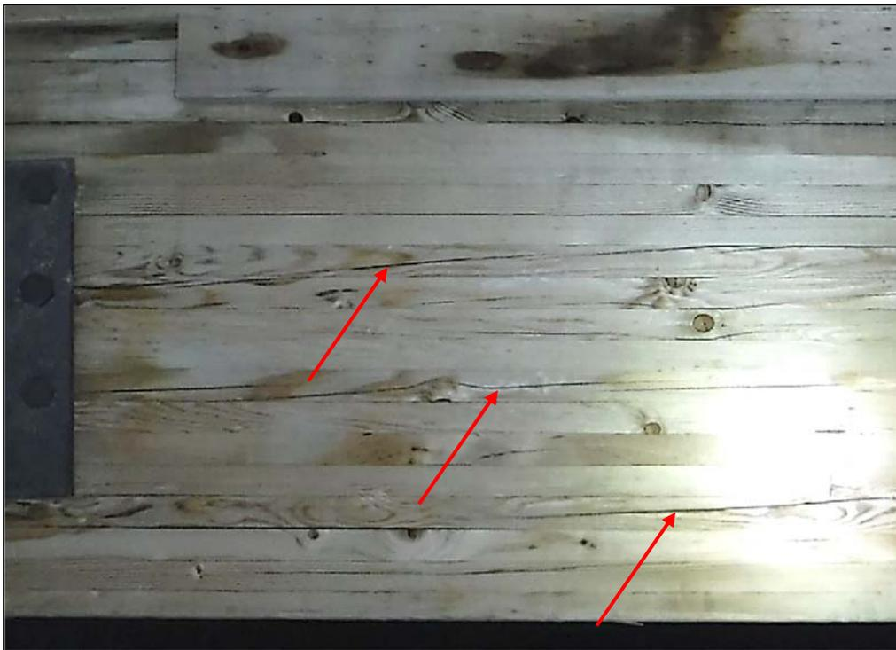
Photo 13 – Close up of the checks seen in Photo 12 pointed out by the red arrows at valley glulam beam 21 between purlins L and K.
