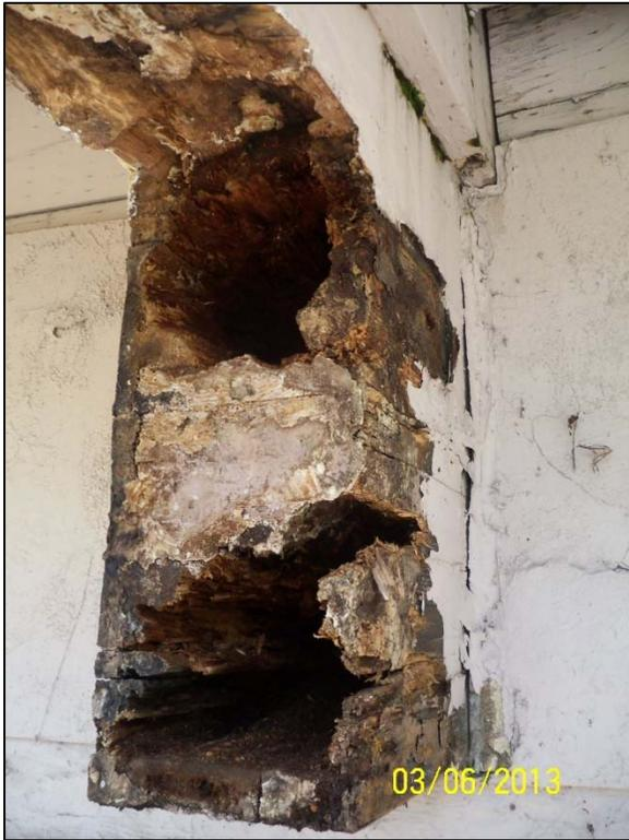
Photo 21 – Valley glulam beam 13 during maintenance repair in 2013, provided by VID staff.
