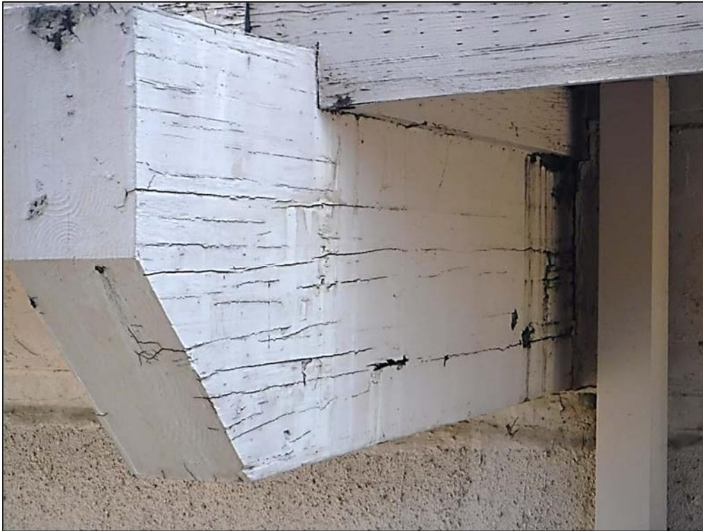
**Photo 14 – Typical dry rot, very soft wood, staining and failed paint found on the exterior portion of valley glulam beam 21.**
