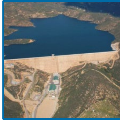
Olivenhain Dam & Reservoir $198 million
