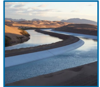
Canal Lining Project $447 million ($190 million from Water Authority)
