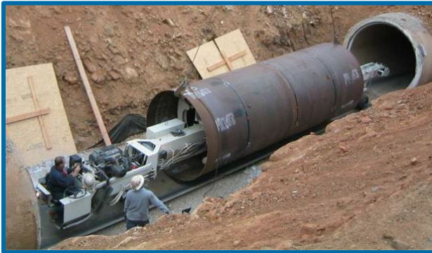
Pipeline Relining $493 million
