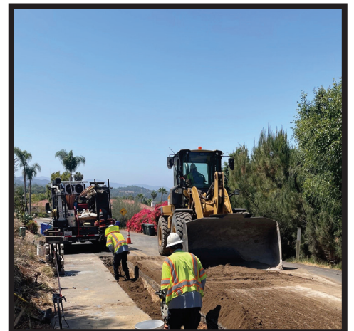
Pictured: Mainline Replacement on Vista Grande
