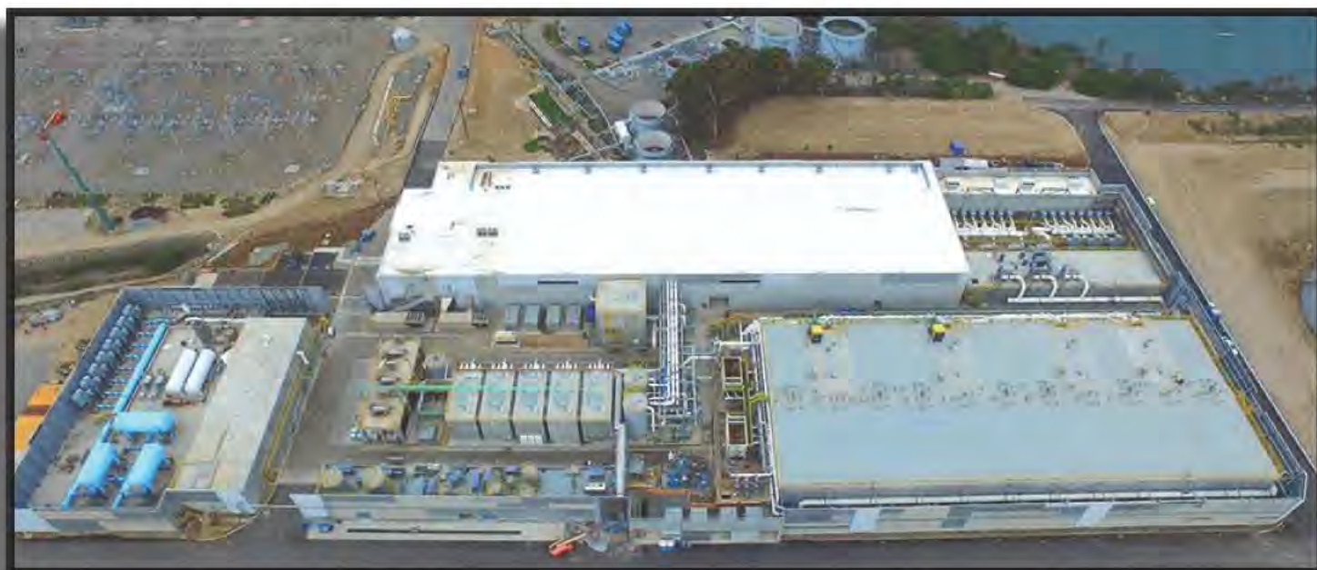
Carlsbad desalination plant. Photo credit: San Diego County Water Authority
