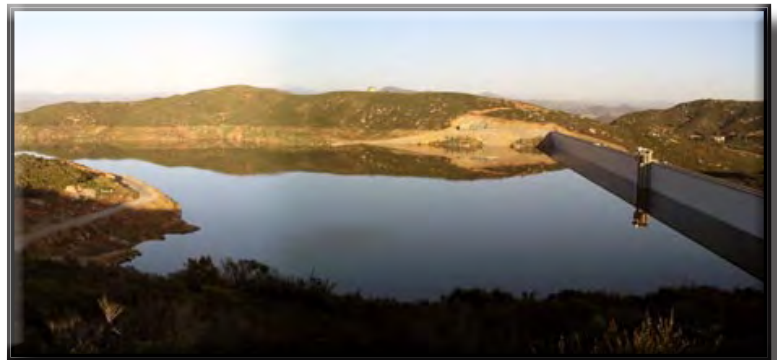
Pictured: Olivenhain Dam and Reservoir Photo credit: San Diego County Water Authority
