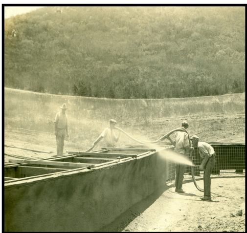
Pictured: Guniting Process on the Flume, circa 1926
