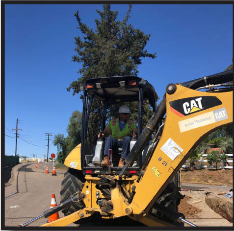
Pictured: Mainline Replacement on York Drive
