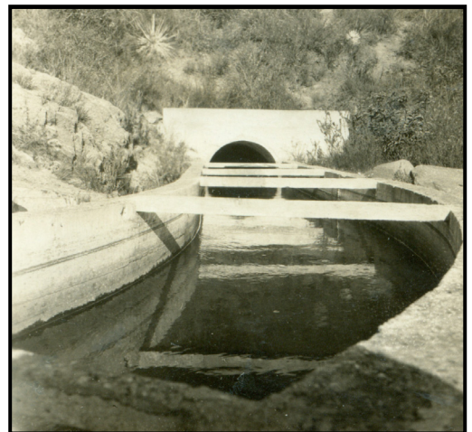
Pictured: Flume exiting Big Tunnel, circa 1930's - 40's
