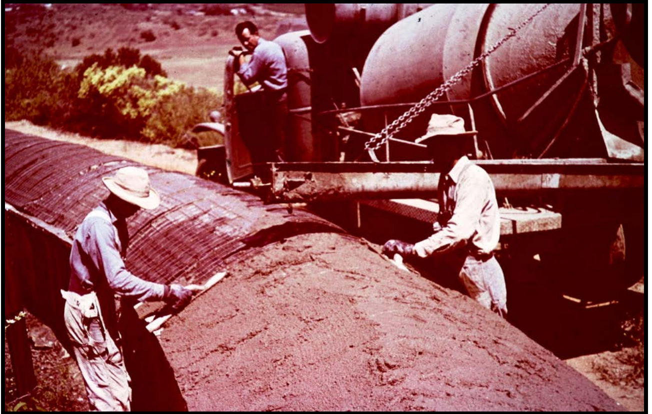
Figure 29: Covering flume cover with hand-placed mortar 1955.
