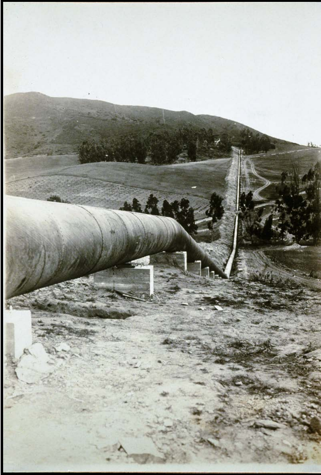
Figure 26: Above-ground portion of Twin Oaks Siphon.
