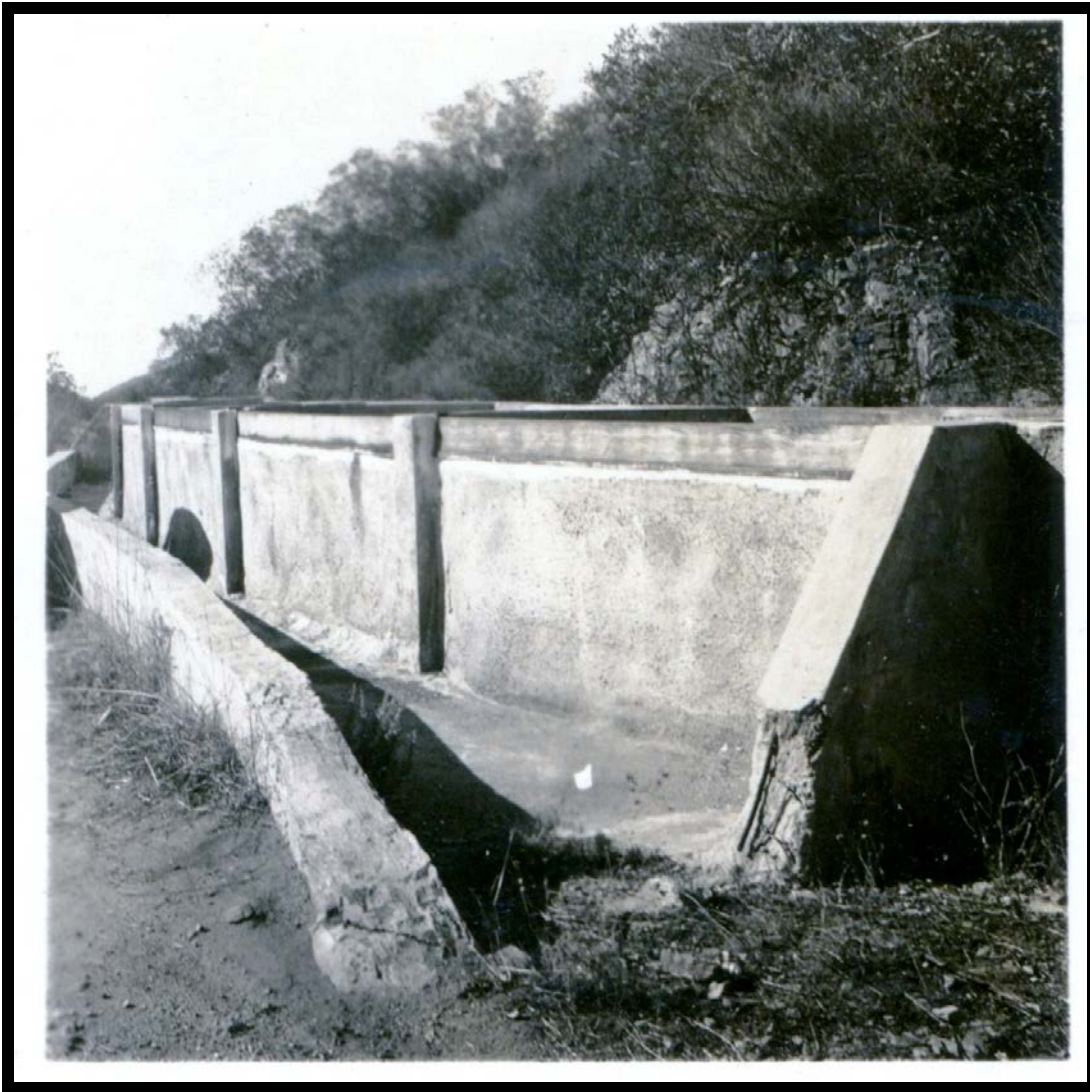
Figure 21: Overflow spillway on Tunnel Bench in the 1930s.
