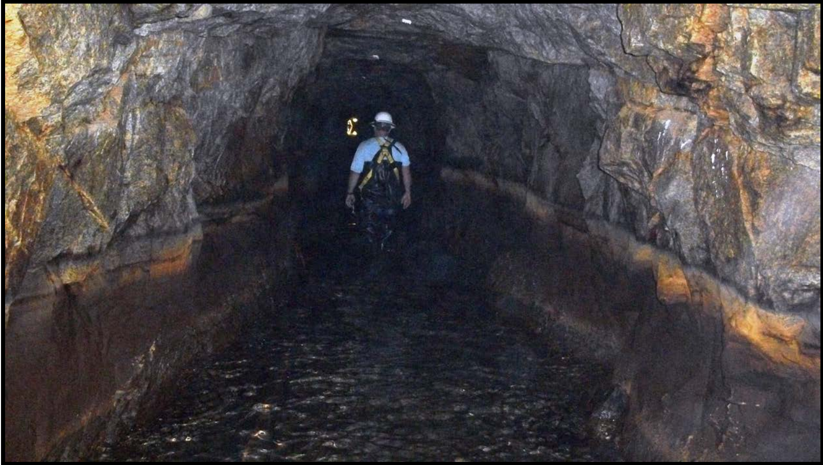
Figure 13: The hard rock interior of Big Tunnel (Tunnel # 2).
