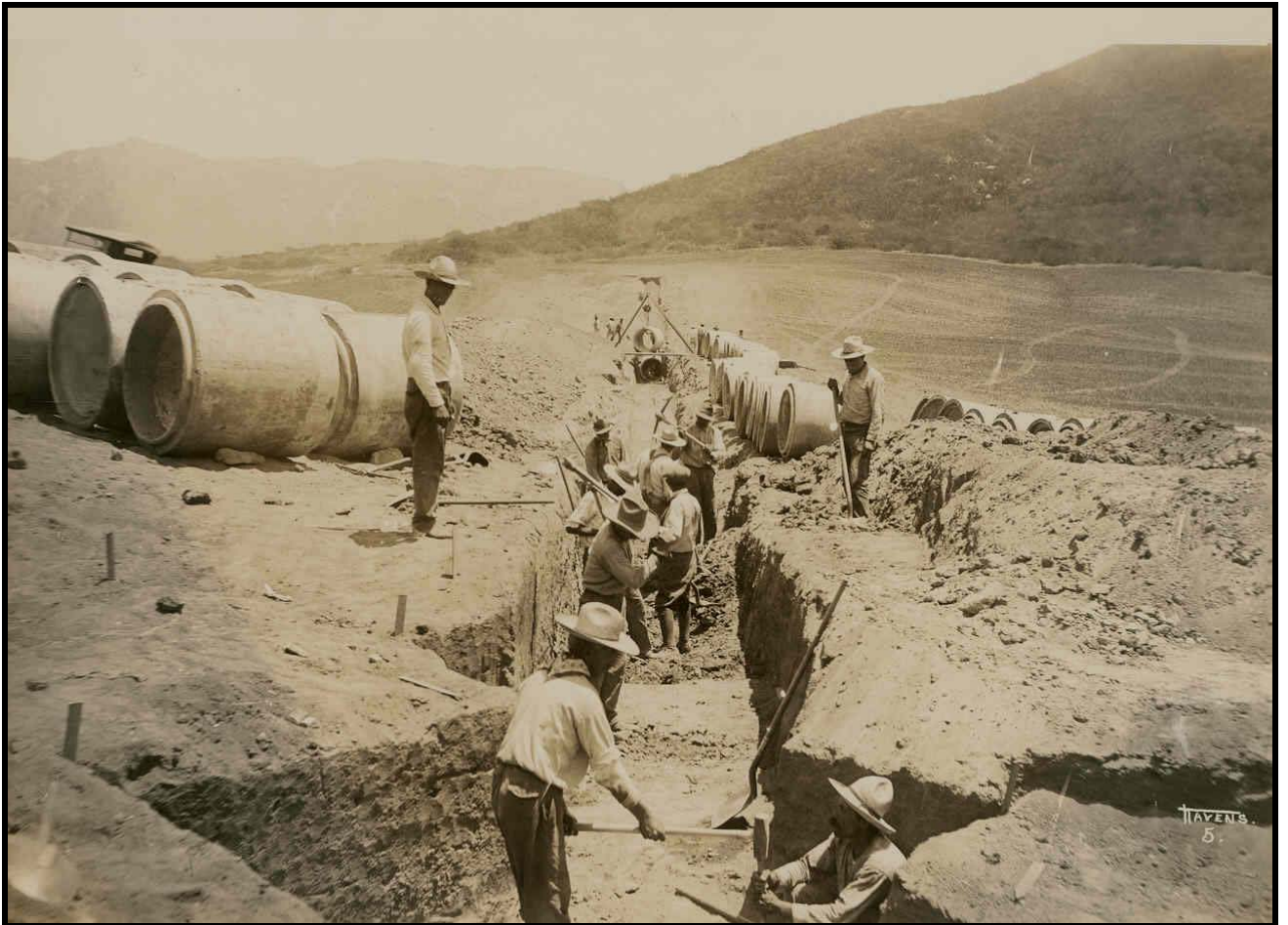
Figure 23: Laying pipe, Caldwell Siphon 1925.
