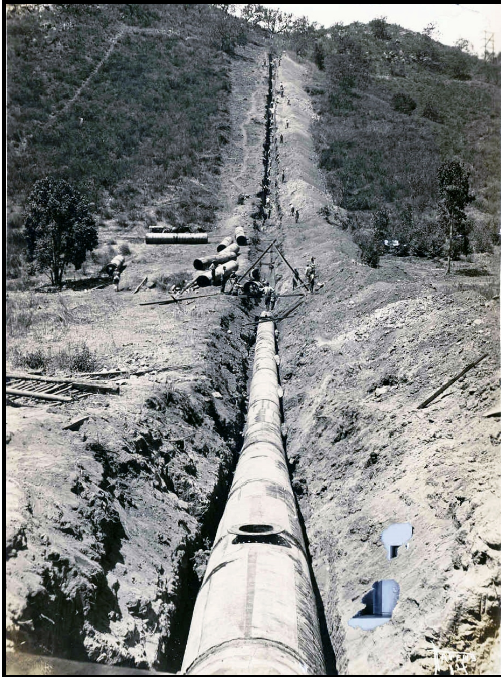
Figure 22: Placing siphon pipe in trench, probably Caldwell Siphon, 1925.
