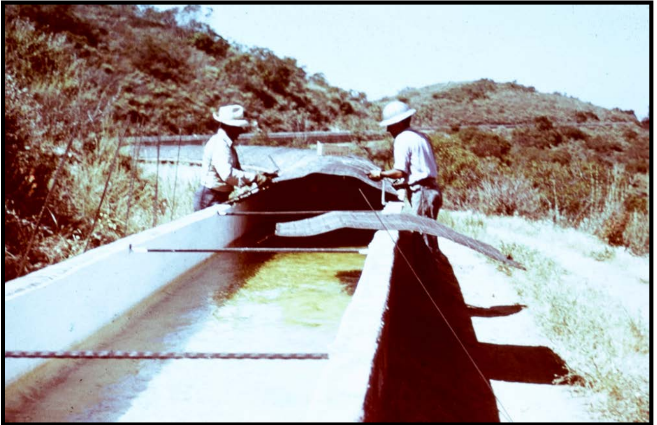
Figure 28: Covering the Flume, 1955.
