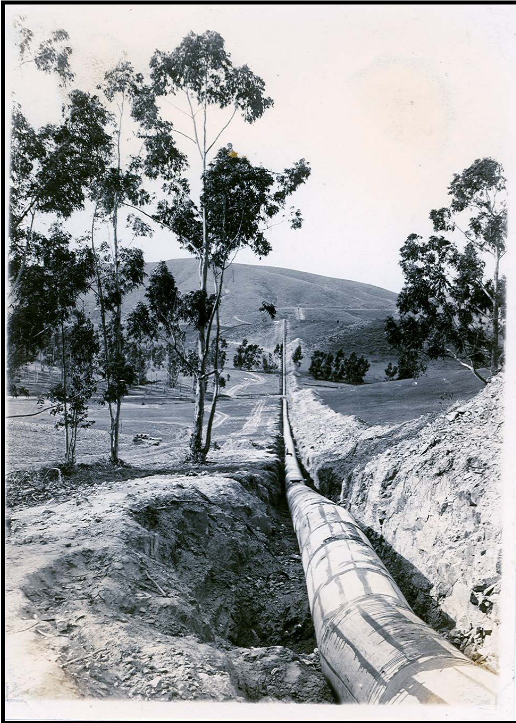
Figure 25: Twin Oaks siphon in trench.
