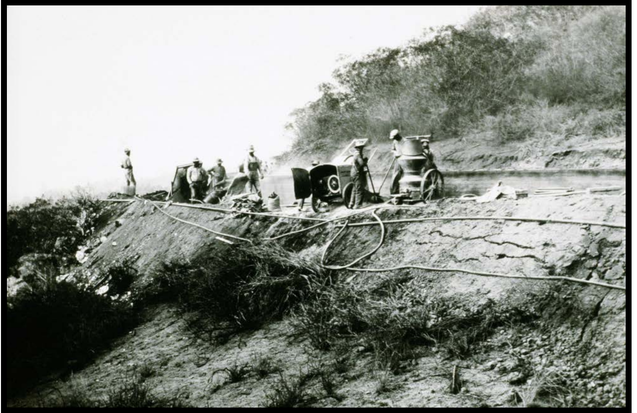
Figure 18: Gunite crew working on flume 1925.
