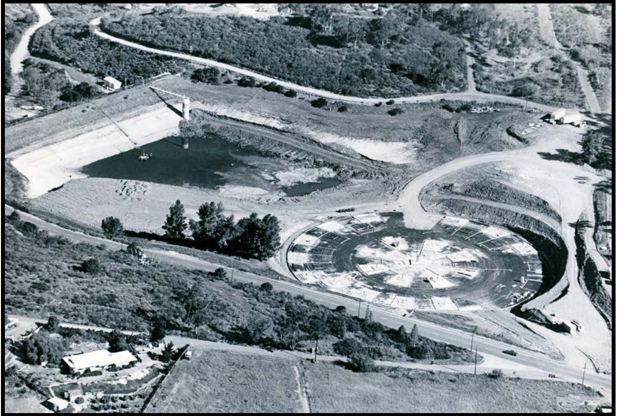
Figure 30: Reconstructing Pechstein Reservoir 1977.
