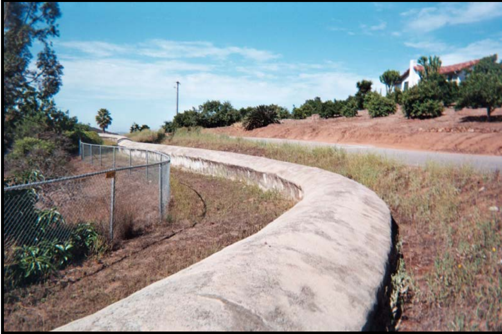
Figure 7: Typical flume section east of Pechstein Reservoir.
