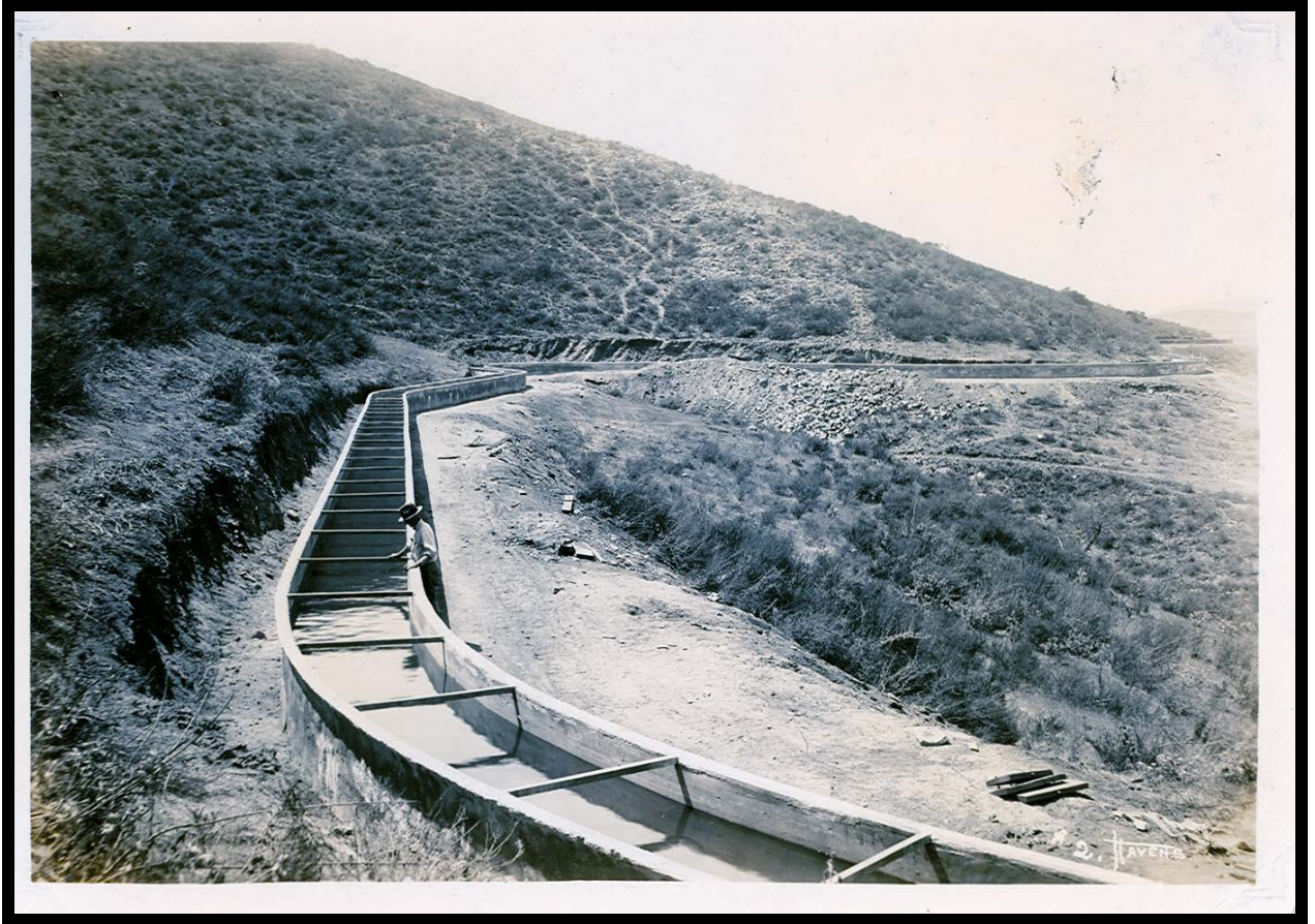
Figure 20: Newly completed Twin Oaks Bench, with water flowing in it.
