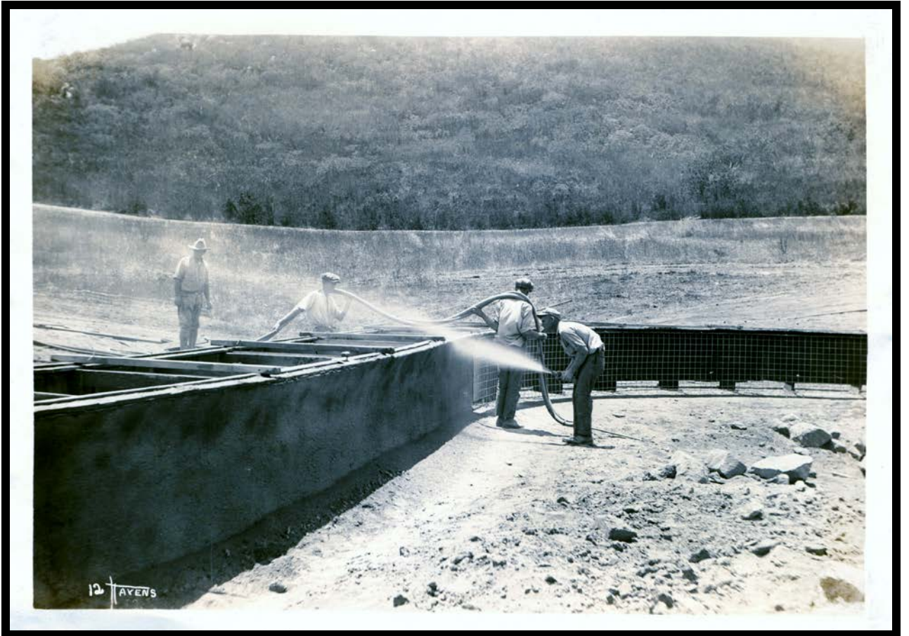
Figure 19: Gunite process at Finkbinder Bench in 1925.
