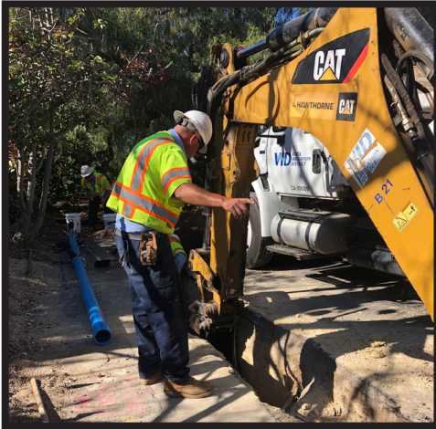
Pictured: Mainline Replacement on Montgomery Drive
