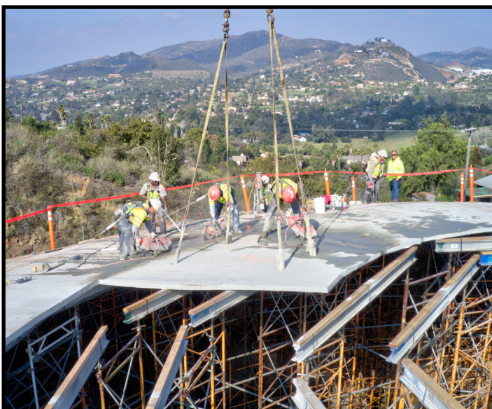
Pictured: HB Reservoir roof demolition in progress
