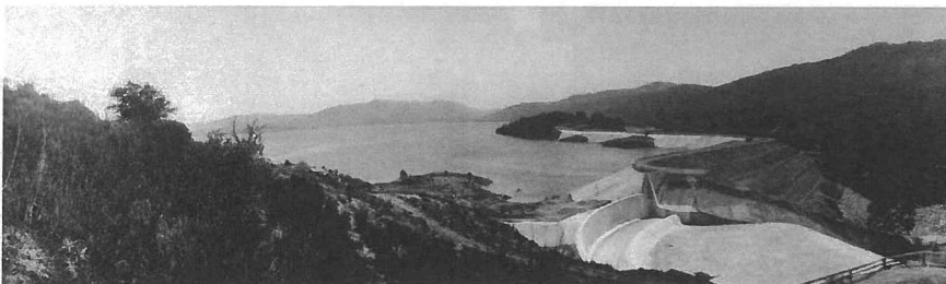
Henshaw Dam April 5, 1928
