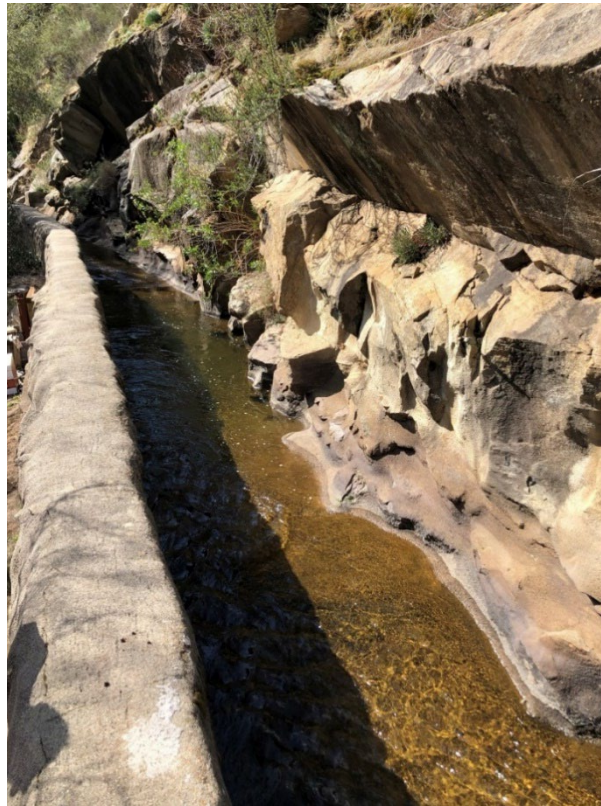
Figure 2-36. Escondido Canal just downstream of the diversion dam, looking upstream, March 4, 2021.
