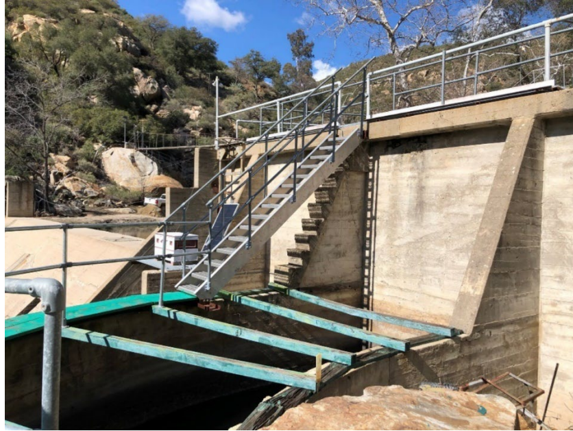
Figure 2-35. Escondido Canal Diversion Dam looking upstream from the right bank, March 4, 2021.
