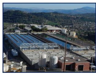
with an on-site chlorine generation system. Project elements included the demolition of gaseous chlorine storage and feed systems, installation of new sodium hypochlorite and chlorine dioxide generation systems, electrical system upgrades and upsizing emergency power generators capable of managing the demands of the redesigned EVWTP. The two newly installed emergency power generators can fully operate the EVWTP during a power outage, thus increasing water supply reliability.
